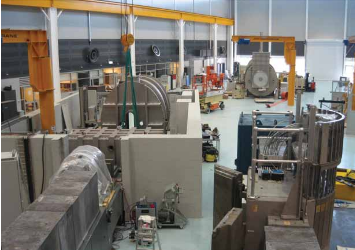
The Neutron Beam Instruments under construction
