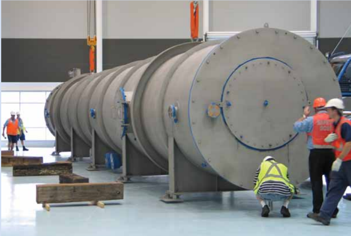
Installation of QUOKKA's vacuum vessel
